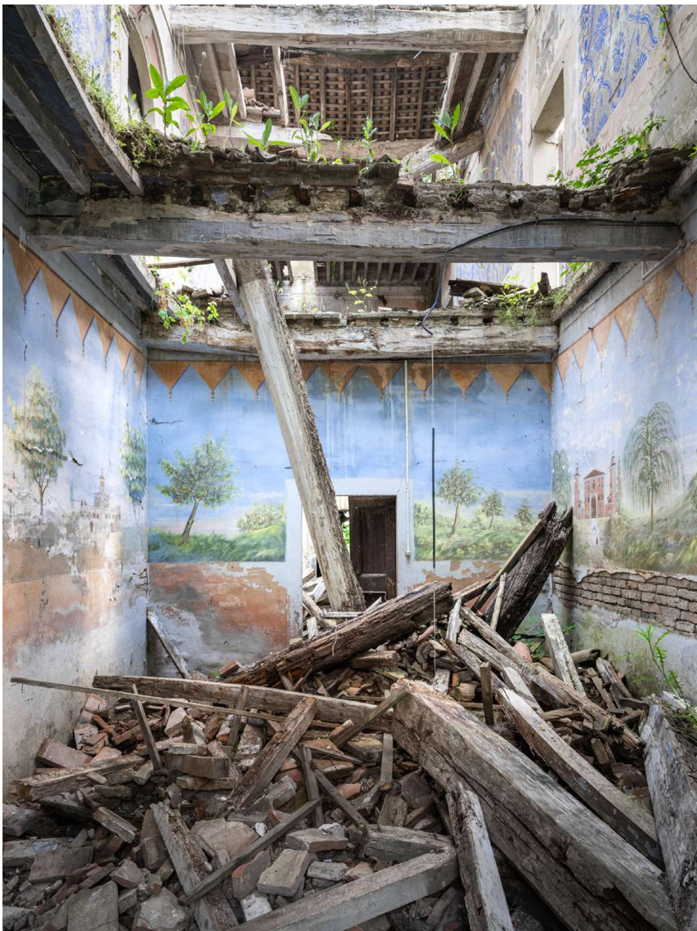
Italy collapsed roof fresco villa interior
