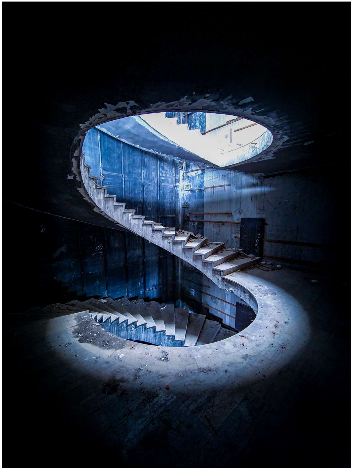
Burned staircase of a former five-star hotel, now just an empty shell with bathtubs stacked in the corridor.
