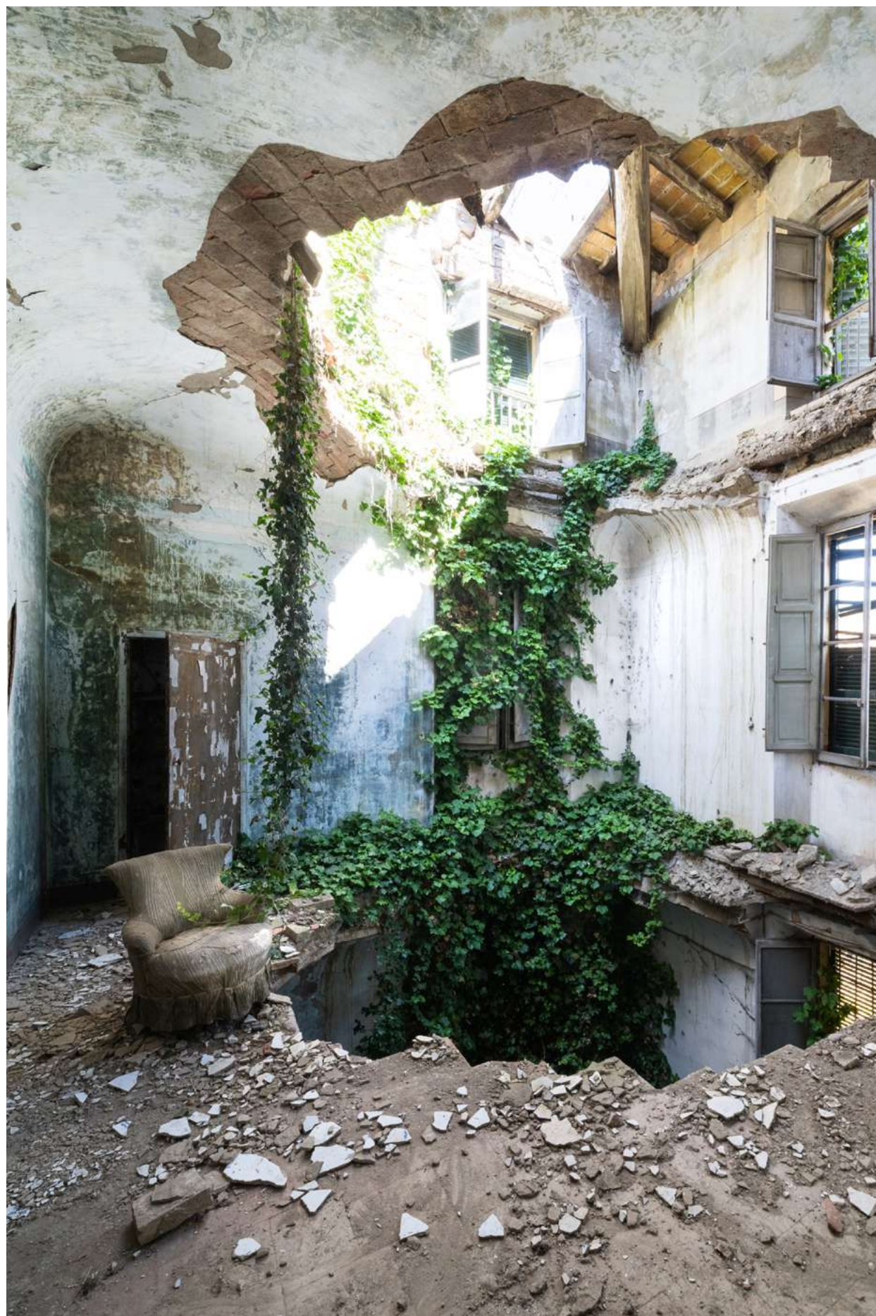
Italy abandoned villa collapsed roof
